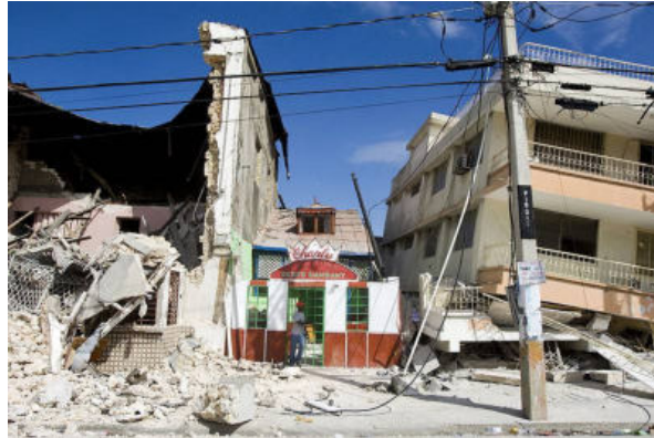
Damaged buildings in Port-au-Prince
